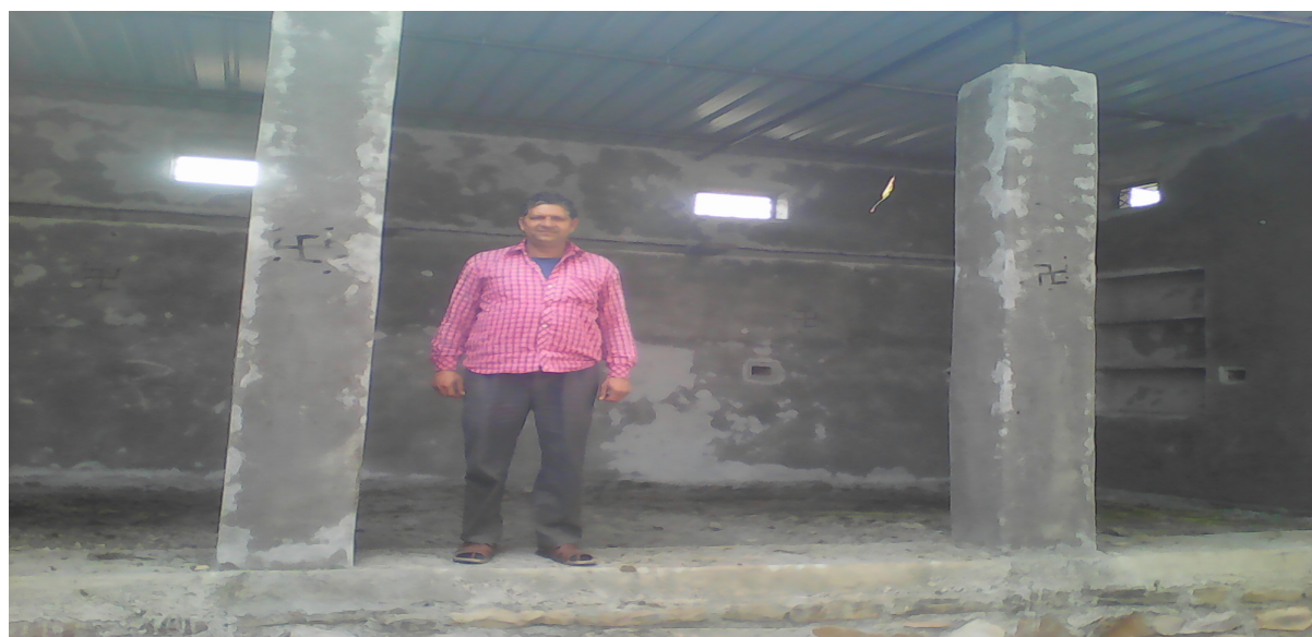
A Beneficiary along with the completed Cattle Shed in Bakani
