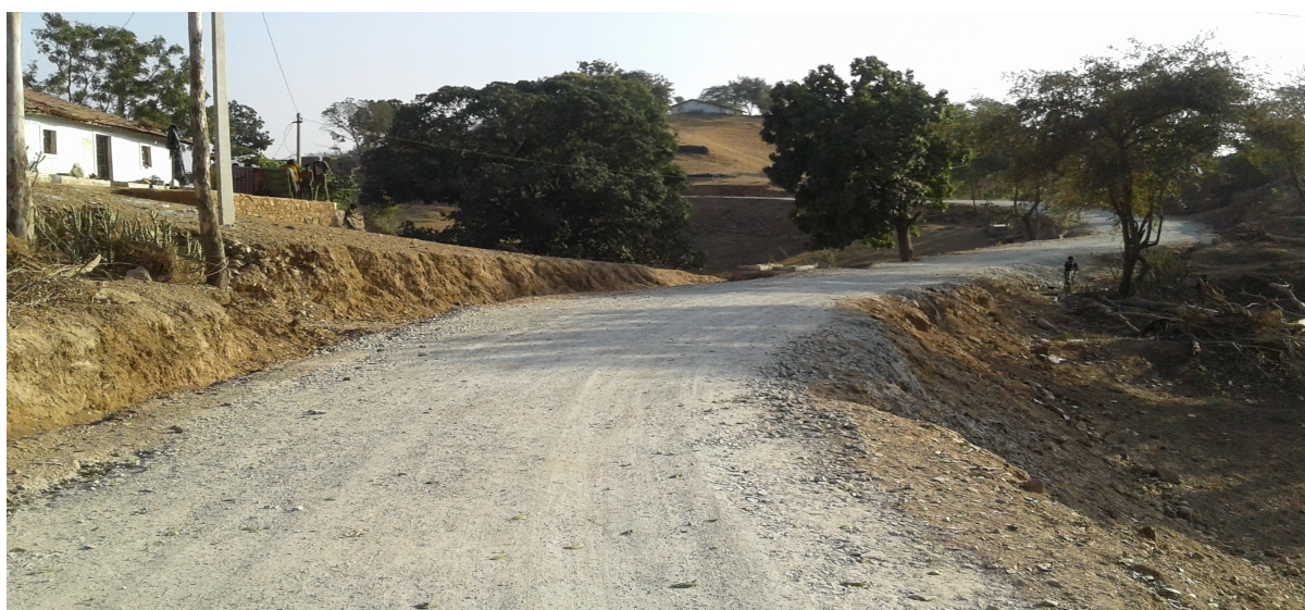
Road constructed under MGNREGA in Jhonthri block.
