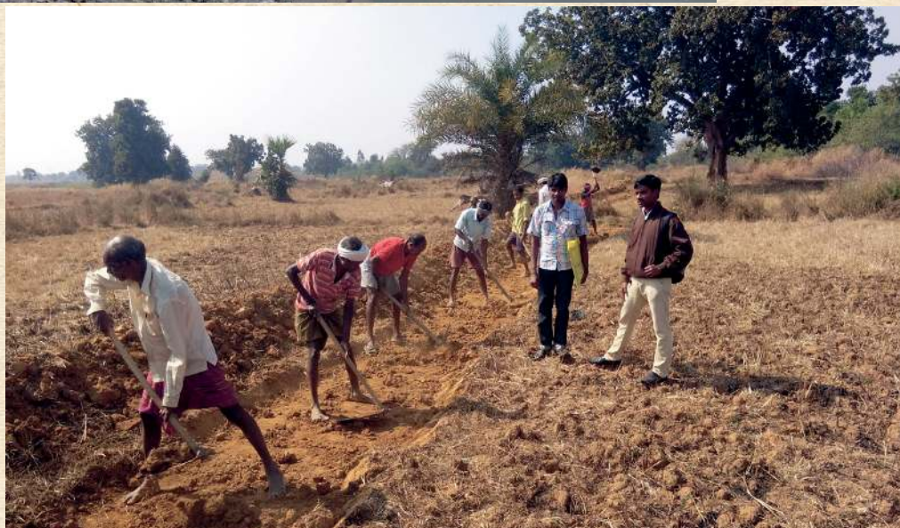
Construction of Farm Bund at Kandhamal, Odisha (SEWA)
