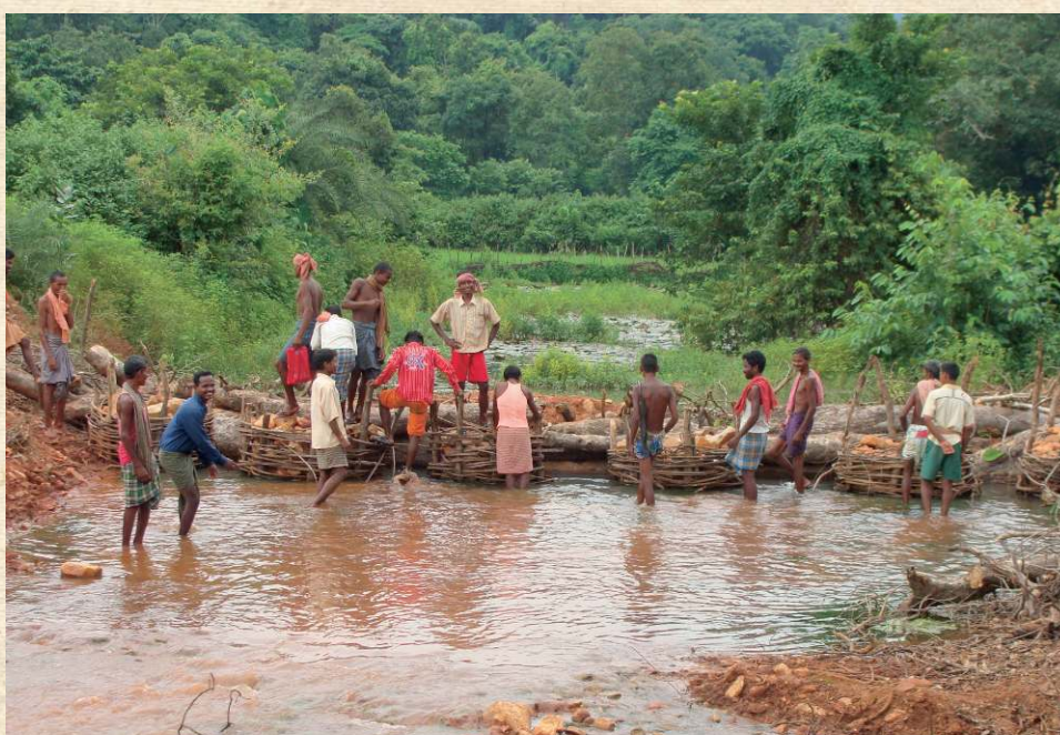
Construction of Brushwood Check Dam: Village: Kalaspur, Panchayat: Balikuma, Block: Kankadahad, Dist: Dhenkanal, Odisha (FES)
