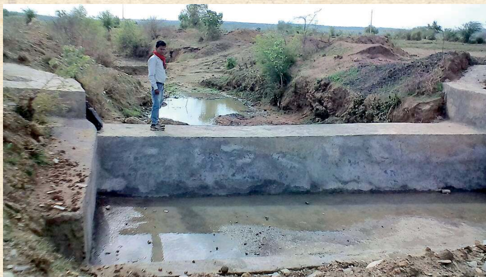
Stone masonry check dam in Shivpuri (Parhit Consortium)
